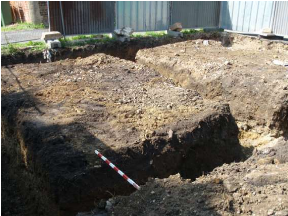
Plate 2. General view of site (looking NW)
