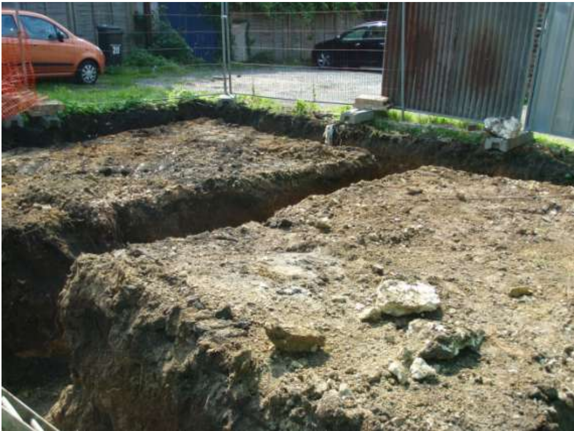
Plate 3. View of trenching (looking NE)
