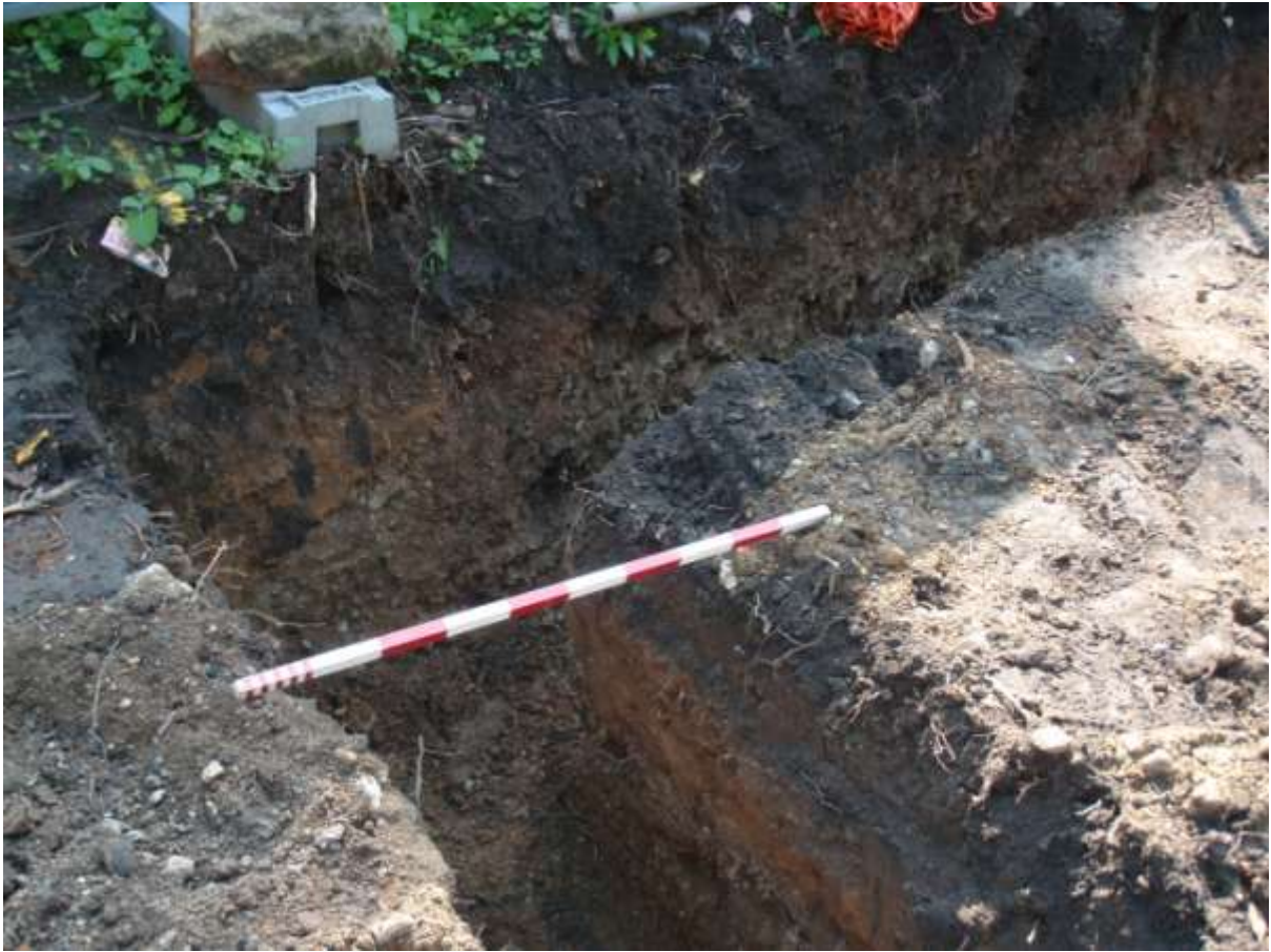
Plate 4. View of foundation trenching (looking SE)
